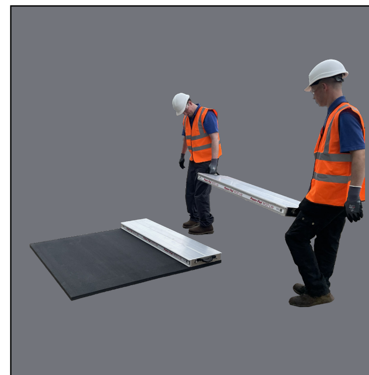
STEP 2 Position the aluminium pads according to the chosen configuration.
