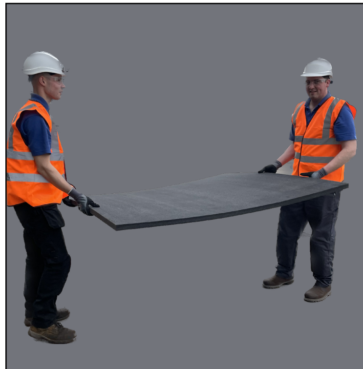
STEP 1 Position 30 mm etha foam (EF700 grade) on firm level ground.
